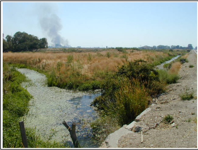
Reach MC:B- View off of County Line Road downstream from Ridenbaugh Canal.
